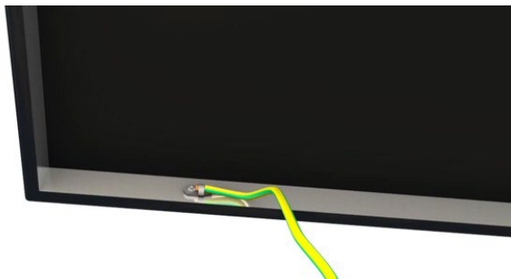
Connection of the ground cable under the pannel
